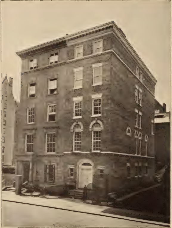
Nos. 20 and 22 West 73d Street.
